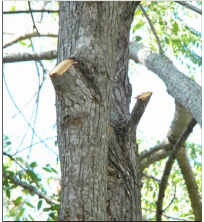
Uneven Cut. These limbs were cut unevenly and they were cut too far away from the branch collar to form a good callus.
